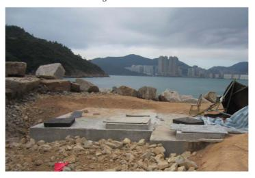
**Photo 2 –** Construction of the new beach manhole has been largely finished, with only small part of backfilling and reinstatement works remaining.
